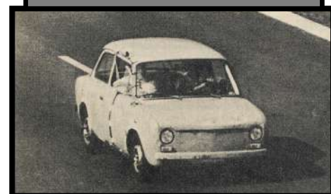
Above and below; 1962-63, the size and the shape of the 2-door car resembles the final product (but still with 1100 type tail lights). Engine is now 4 cyl, 850 cc.
